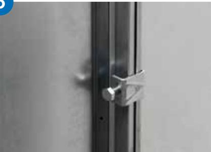
Assemble the Rectangular Joint Bolt Clamp RJBC over the flanges.
