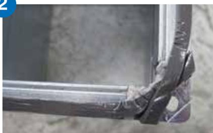
Apply the seal moulding (RJSM) to the outer edge of the connection profile.
