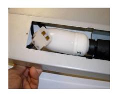
Figure 9: Passing cable through
